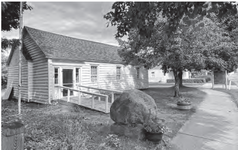
The historic Schoolcraft house on the east end of Water St. in Sault Ste. Marie, Mich.
