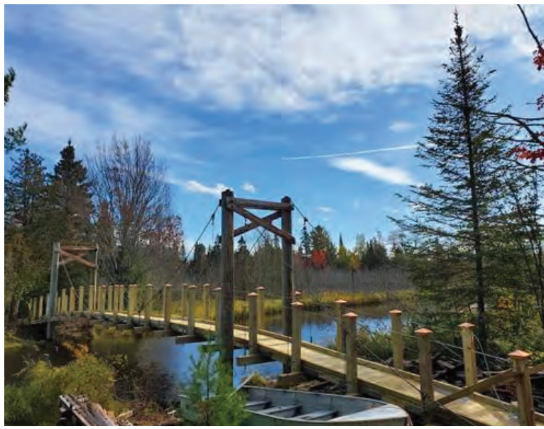
The new Naomikong Bridge was completed in September.
