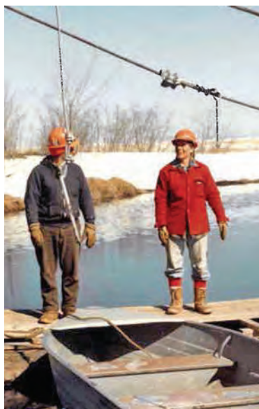
Naomikong Bridge during construction in the 1980s.
