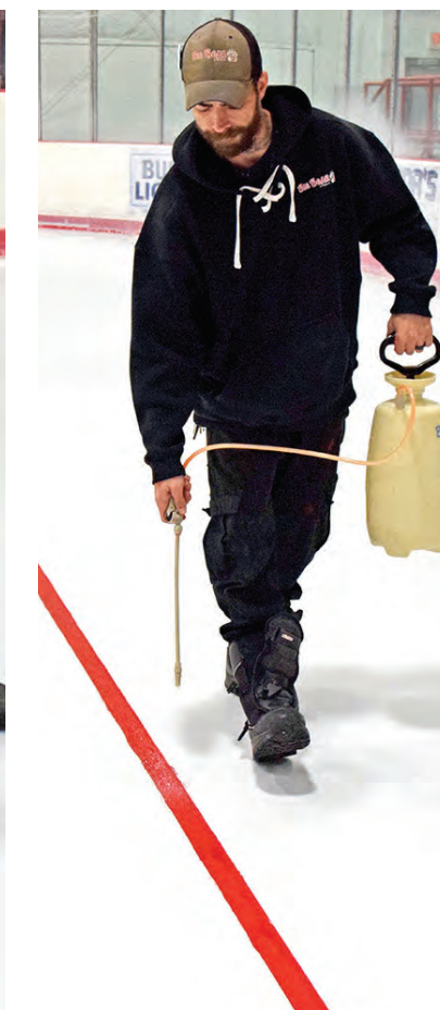
Chris Gurnoe uses specialized equipment to "freeze-in" the goal line after painting to perfection.
