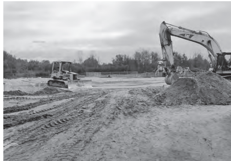
Site preparation, Wednesday, Oct. 7.
