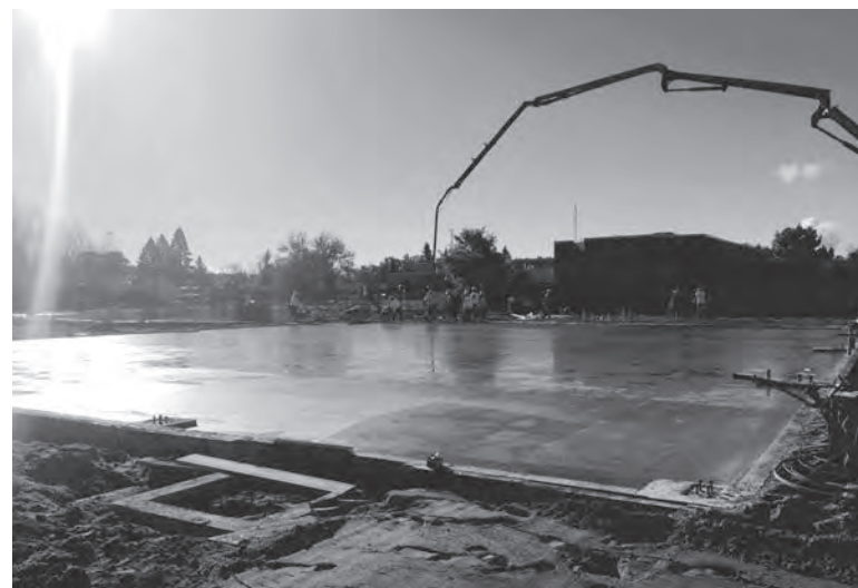
Finishing up pouring concrete the evening of Oct. 7.
