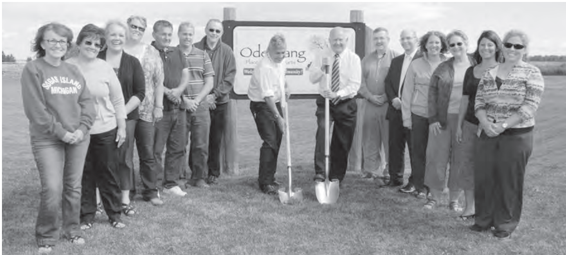
Sault Tribe Chairman Aaron Payment (left center) and Mayor Pro-Tem Bill Lynn manned shovels on July 23 at a ceremonial groundbreaking bringing city water service to the Odenaang Subdivision. The joint venture brought out Sault Tribe Unit I Director Kim Gravelle, Housing Commission Vice Chair Shirley Goudreau, Housing Director Joni Talentino, project specialist Joanne Umbrasas, Unit I Director Denny McKelvie, site engineer Jeremy Gagnon and Chairman of the Sault Tribe Housing Authority and Housing Authority Unit II Representative Ken Ermatinger, the city was represented by Commissioner Don Gerrie, City Manager Oliver Turner, Commissioner Kathy Twardy, Commissioner Pat Shimmens, city clerk/assistant city manager Robin Troyer and city engineer Linda Basista.
