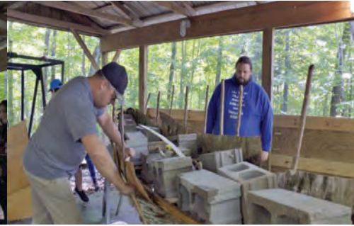
Putting stakes in the frame.
