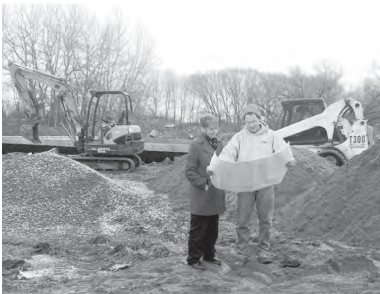
Superior Health Support Systems President Tracey Holt and Dan Arbic of Arbic Construction look over plans for a six-bedroom, 3,000-square foot home for dementia patients under construction on Hyde Street in Sault Ste. Marie, Mich. Details regarding naming opportunities will be announced in February.
