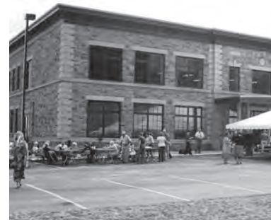
The 92-year-old completely restored building, at 622 W. Superior, will fulfill the needs of area tribal members.
