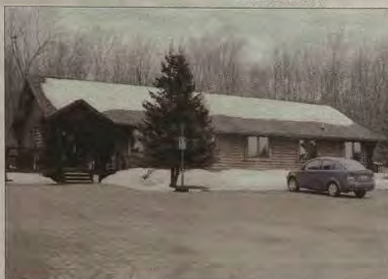
The former Munising Health Center.
