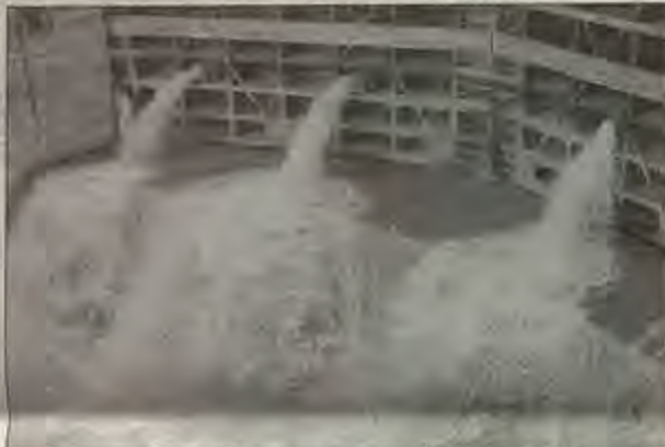
Taken prior to the Poe Lock opening for the season on March 25, four ice clearing culverts pour tons of Lake Superior water over the debris pit from the newly repaired lock gates.
