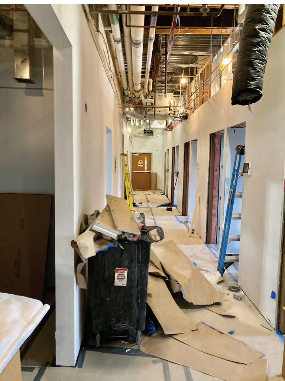
Hallway in the midst of renovation
