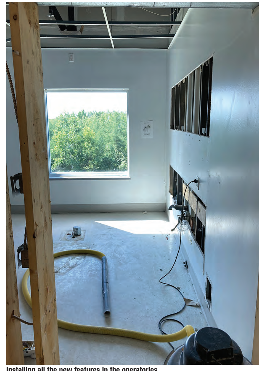
Installing all the new features in the operatories.
