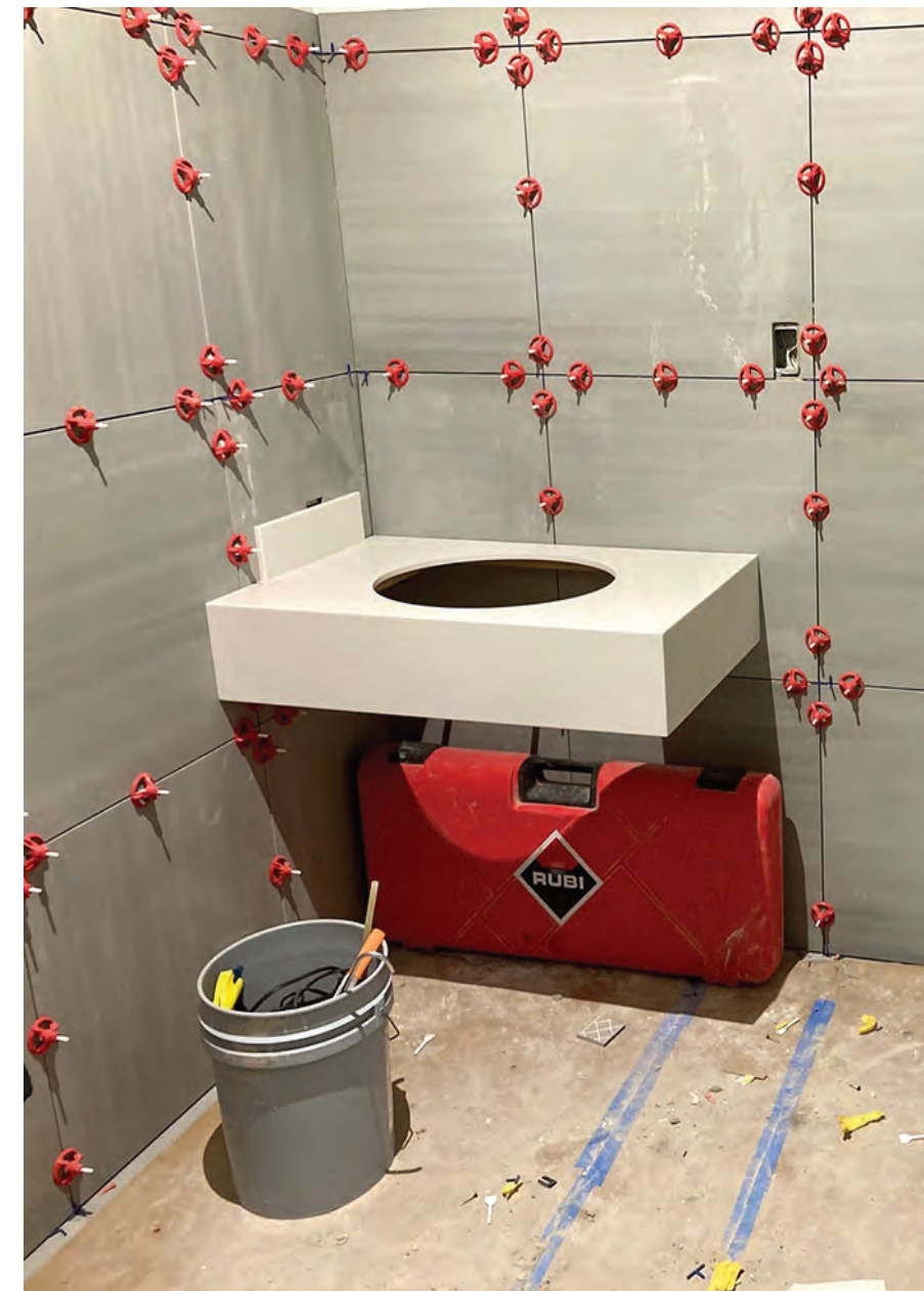
New bathroom going in.
