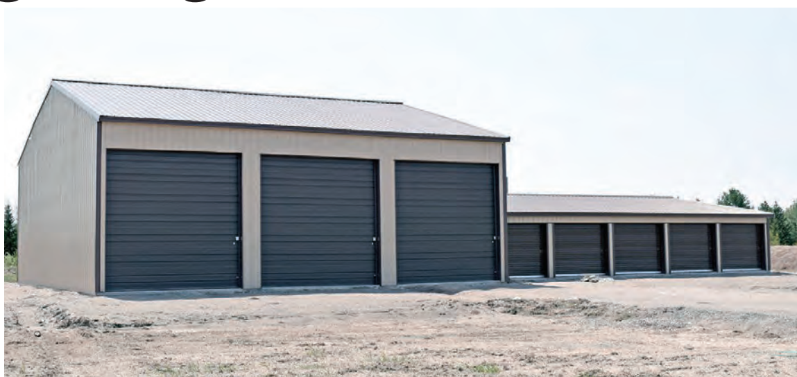
The tribe's new storage facility, located at Odenaang.
