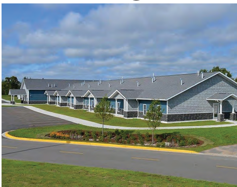
The completed Shirley Goudreau Elder Complex in St. Ignace.
