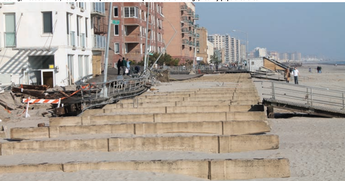
Boardwalk in Belle Harbor along the Atlantic Ocean ripped from its anchorages and pushed against buildings along the beachfront.
