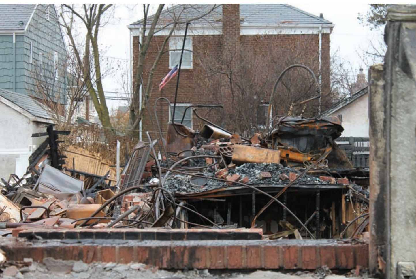
Remains of one of the many homes in Belle Harbor, N.Y. destroyed by Superstorm Sandy. The storm not only brought high winds and flooding, it caused fires, heavy sand deposits and other problems over a large, heavily populated area.
