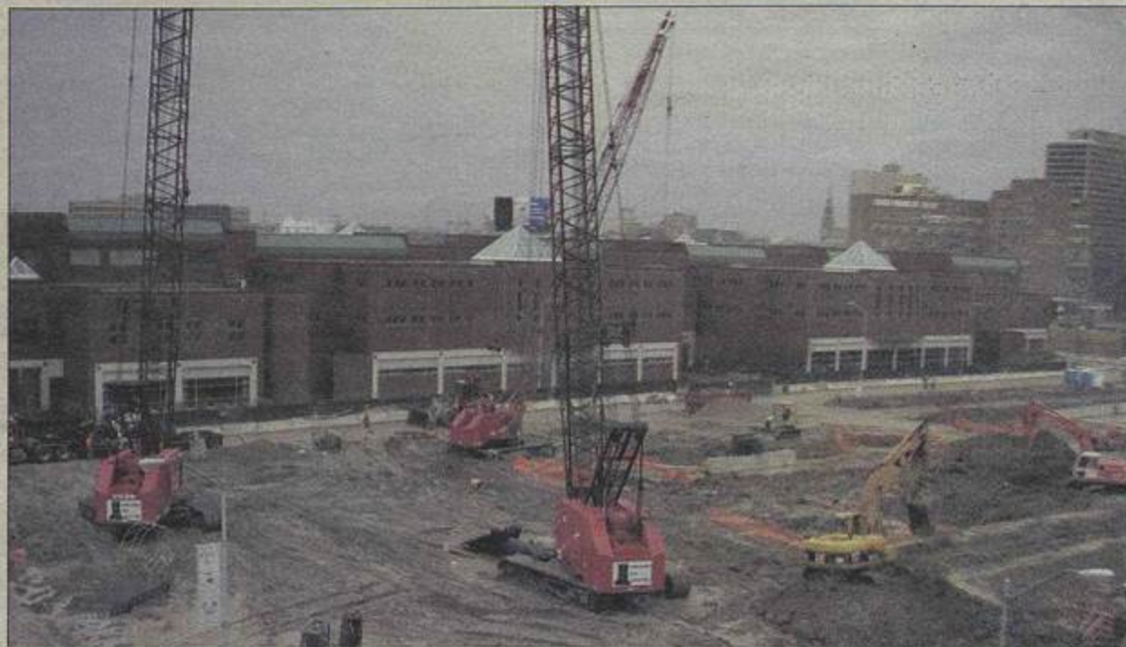
Construction crews work to finish the foundation for Greektown Casino's permanent parking structure. The parking garage and pedestrian walkway connecting the structure to the casino are scheduled to open on time in fall 2007.
